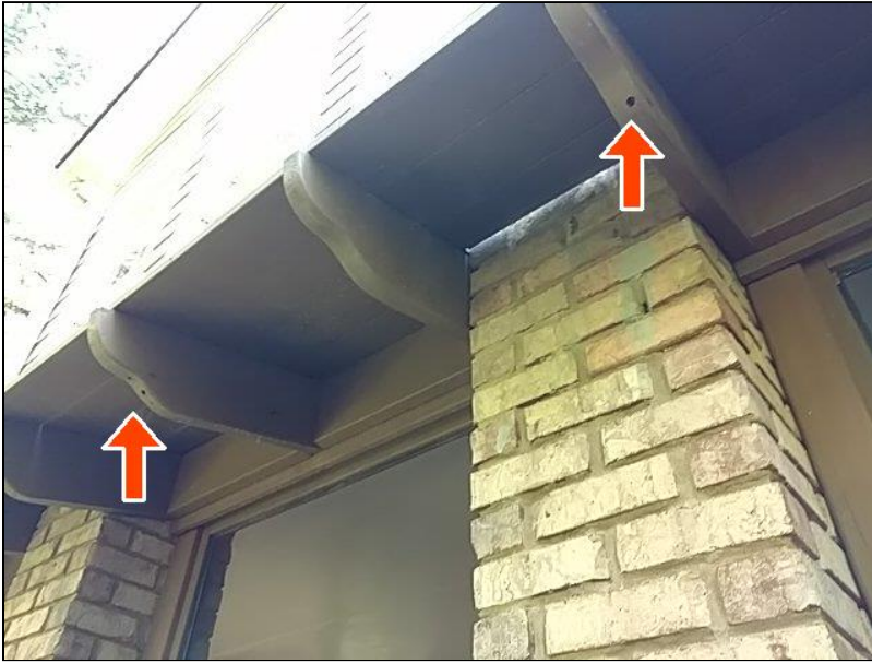
Rear right portico/roof
