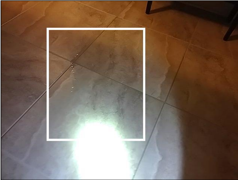
Rear left basement
