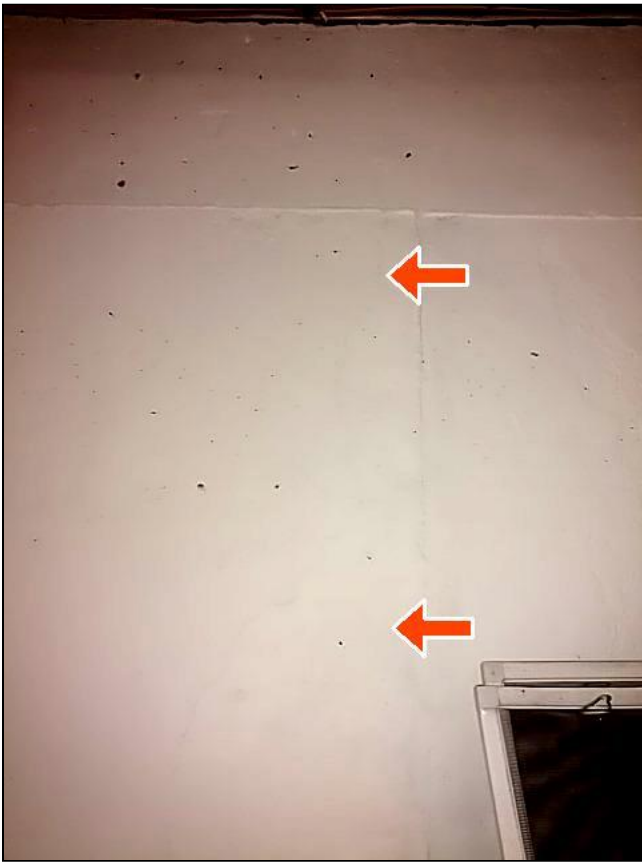
Front basement wall
