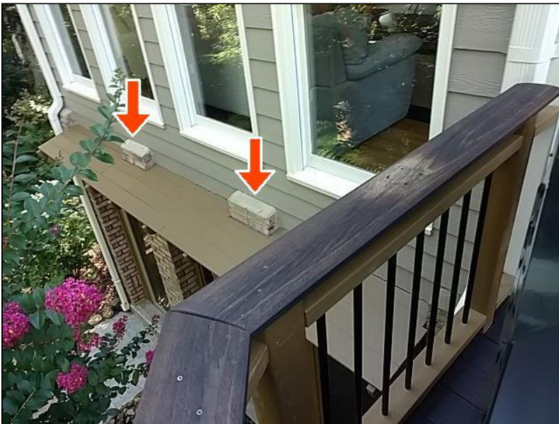
Rear right columns
