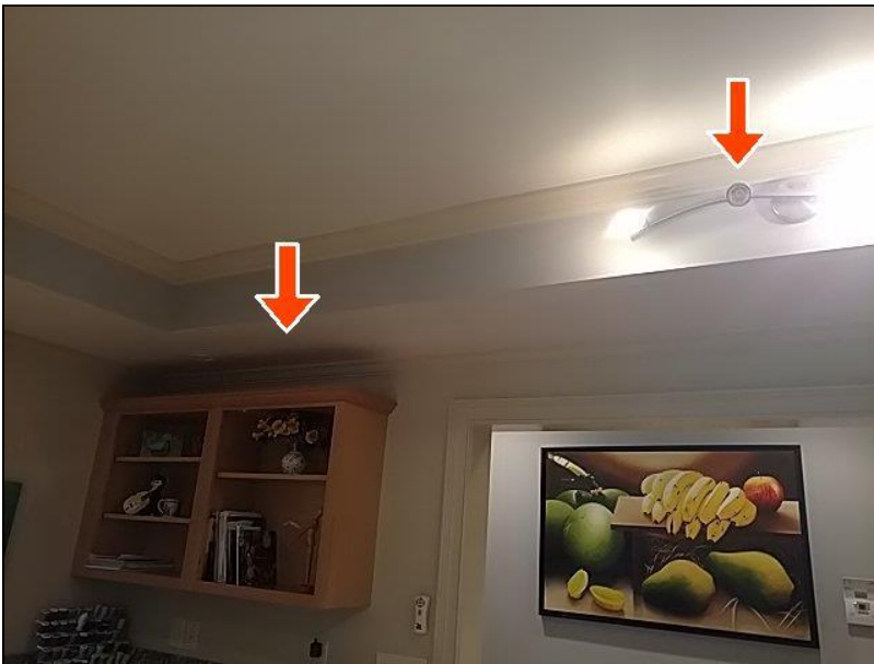
Rear center basement
