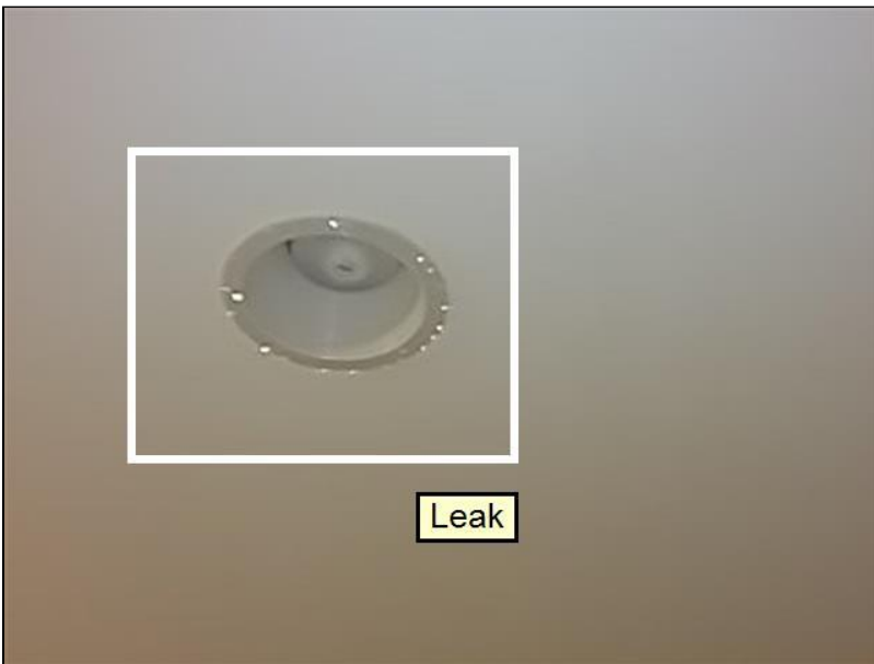
Rear left basement
