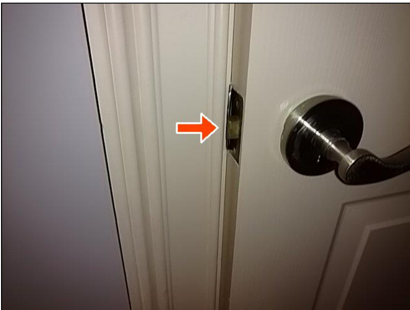
Rear left basement
