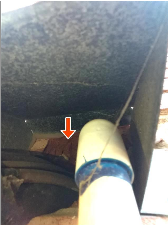
Wall penetration at left
